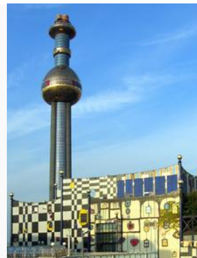
Spittelau incineration plant in Vienna
